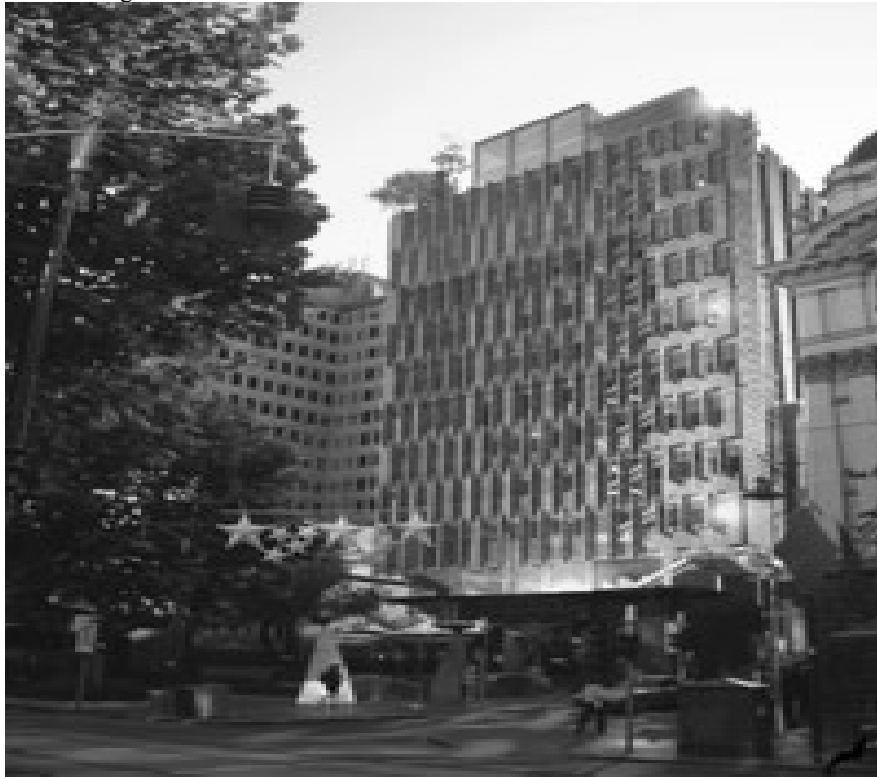
Fig. 7 Council House 2 (CH2), Melbourne, Australia. by Architect Mick Pearce. Source: [2]
