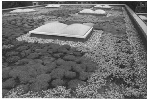
Fig.5 Typical green roof. Planted roof preserve the site putting back into the environment the nature the buildings remove. Source [17]
